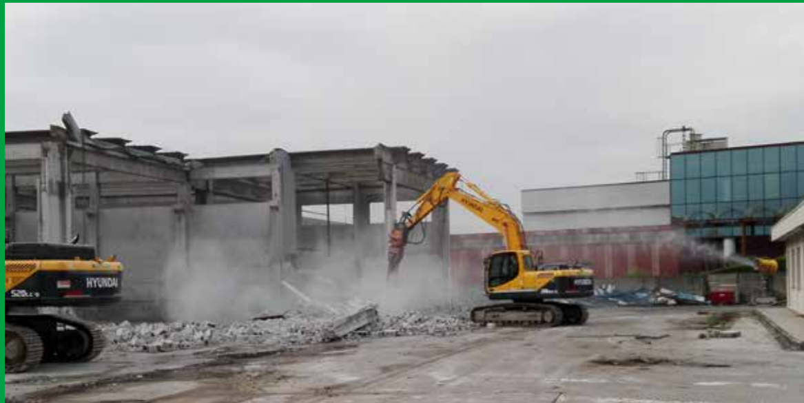
SITE IN NUMERIA – SAN FIOR (TV) - BEGINNING OF WORKS
